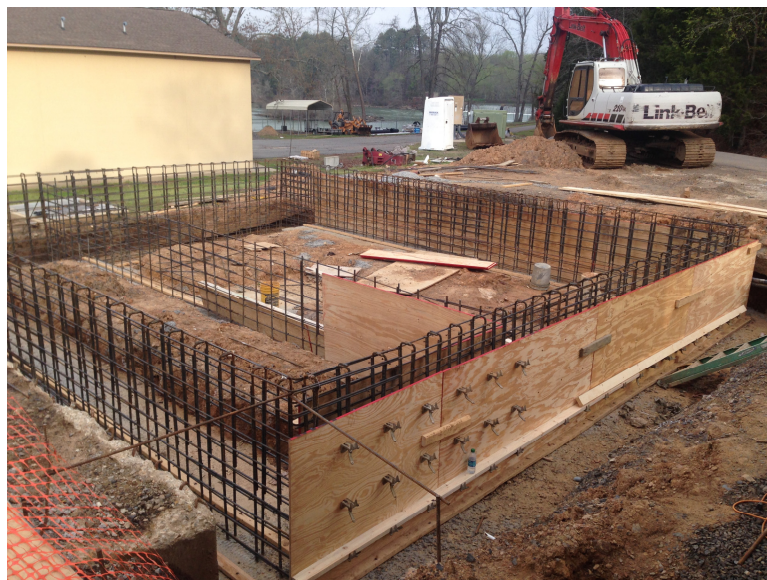
April 1, 2015 – Placement forms for stem walls.
