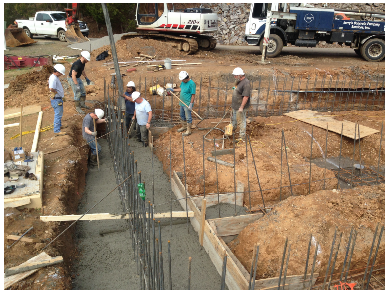
March 19, 2015 – Placement of concrete for Alum Building foundation.
