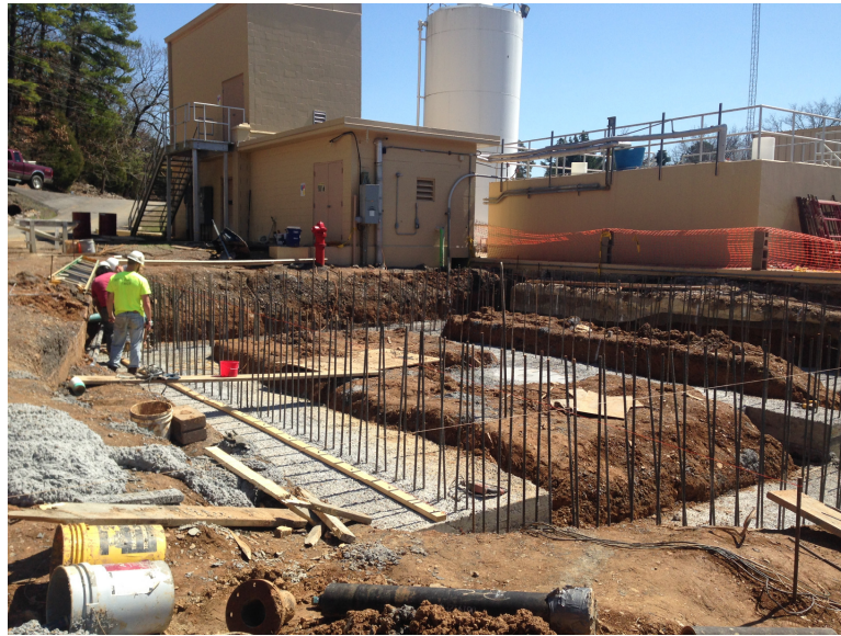
March 23, 2015 – Placing reinforcement / rebar for the stem walls on the new foundation.
