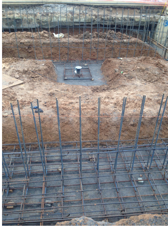
March 18, 2015 – Removal and replacement of reinforcement and trench soils due to weather conditions.
