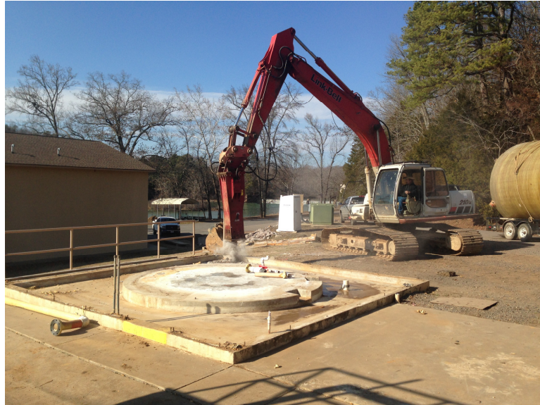
January 23, 2015 – Existing alum building foundation demolition
