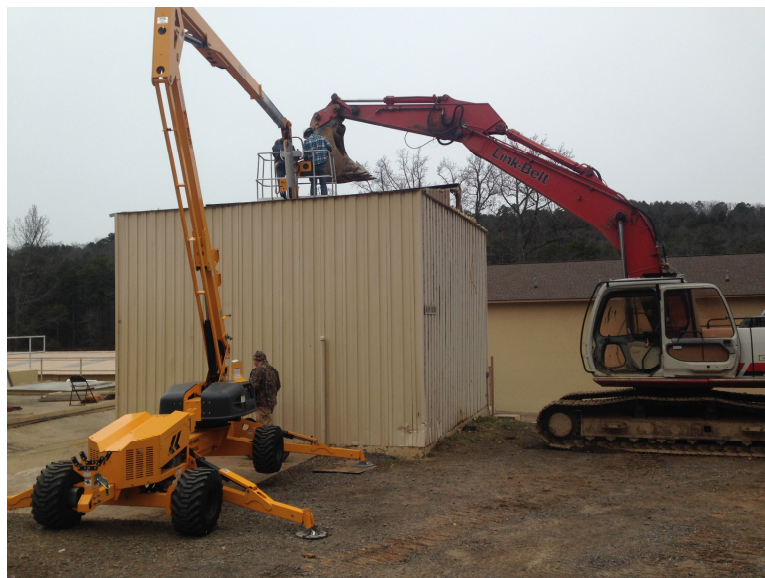
January 22, 2015 – Demolition of existing alum building
