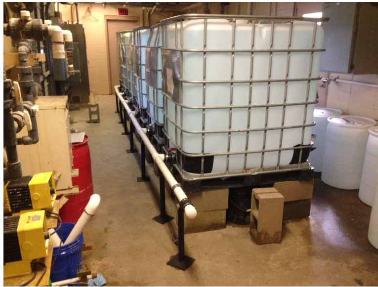
January 14, 2015 – Temporary alum storage and feed system
