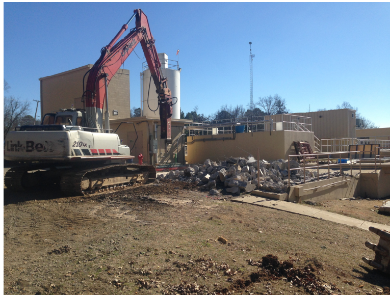
January 26, 2015 – Existing alum building foundation demolition
