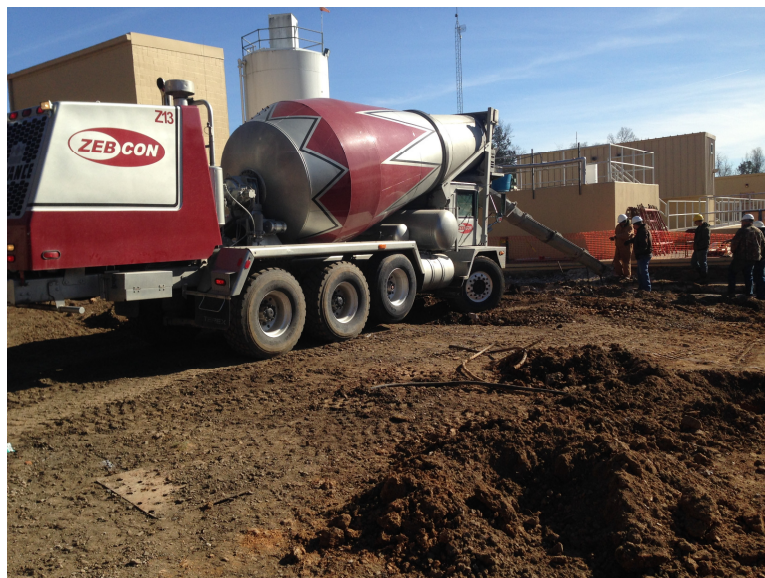
February 2, 2015 – Placement of flowable fill under old influent trough
