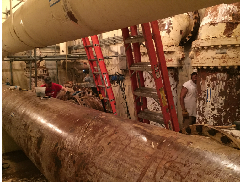
June 9, 2015 – Cleaning of the piping and other prep work for the painting of the plant filter piping gallery.
