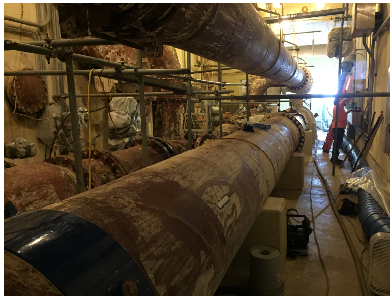
June 18, 2015 – Prep work for painting inside the pipe gallery.
