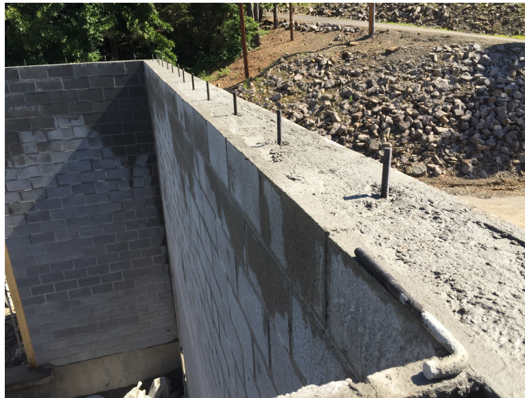
June 10, 2015 – Placing reinforcement and filling cells with grout for the construction of the walls including the bond beams with J bolts on the new alum building.
