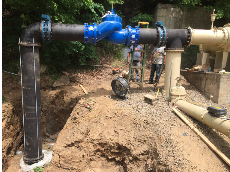
June 17, 2015 – Installing new 18" DI flange T, butterfly valve and FL x PE spool piece.
