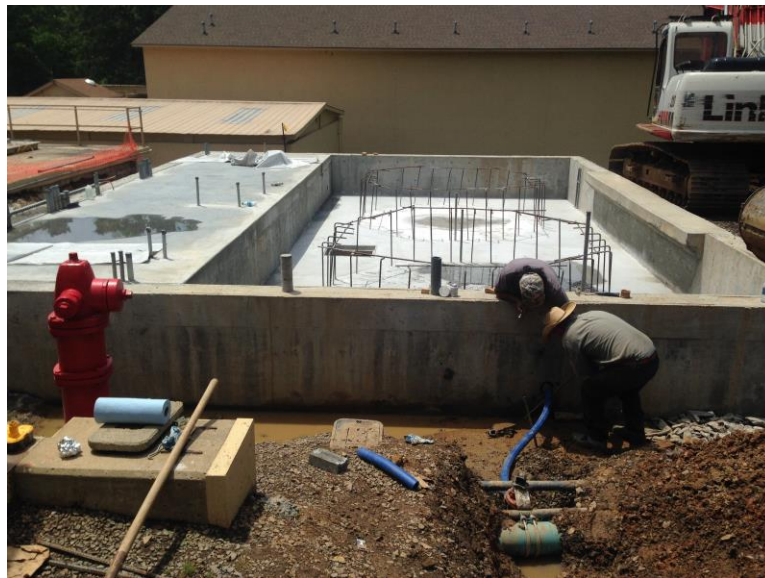
May 15, 2015 – Making a tap on the existing 6" PVC water main and install 2" valve and piping for the water service to the new alum building.
