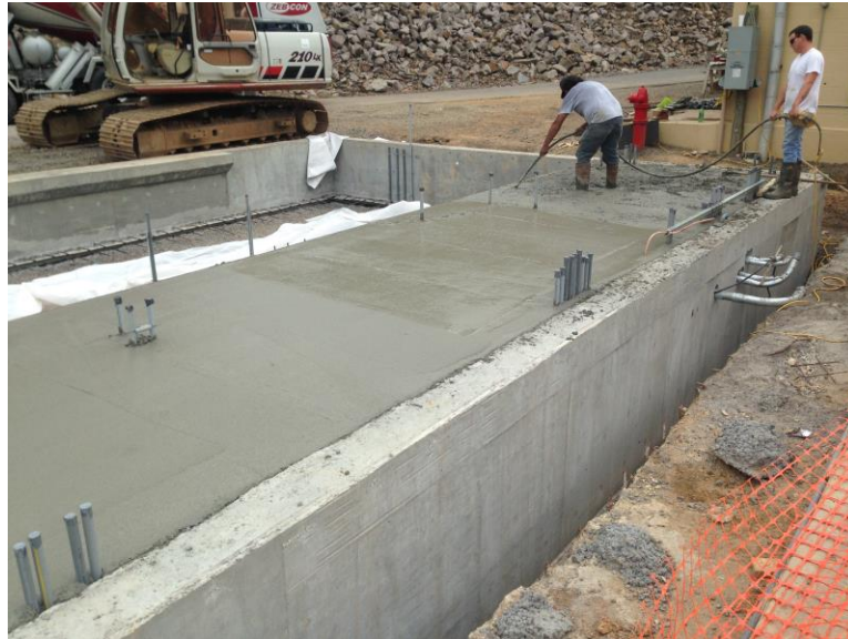
May 7, 2015 – Placing concrete for the south half floor slab of the new alum building.
