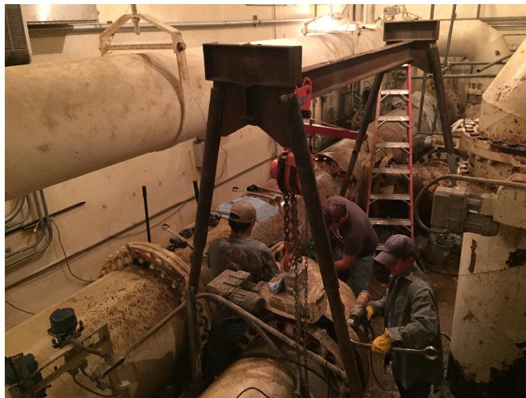
May 28, 2015 – Installing new 24" butterfly valve and actuator in the WTP filter piping gallery.
