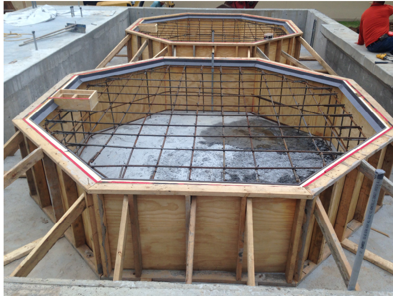
May 21, 2015 – Concrete forms and reinforcement for the bulk storage tank foundation pads in the new alum building.
