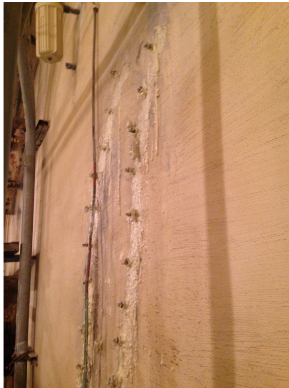
March 6, 2015 – Grout installation to seal small cracks in the walls
