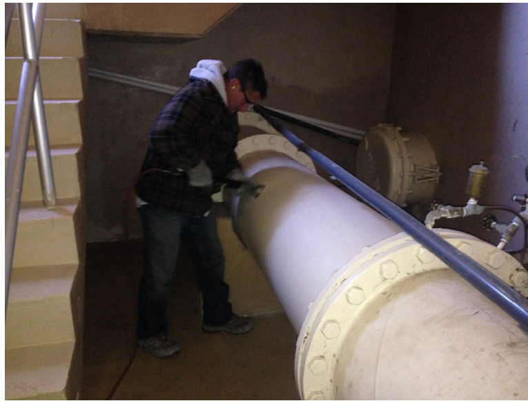
February 18, 2015 – Preparing wall thickness testing locations in the pipe gallery
