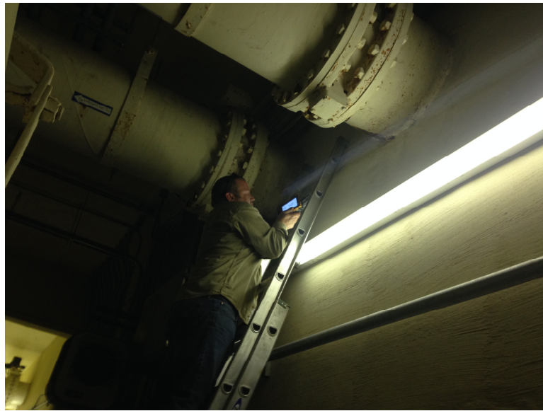
February 25, 2015 – Performing wall thickness testing on pipes
