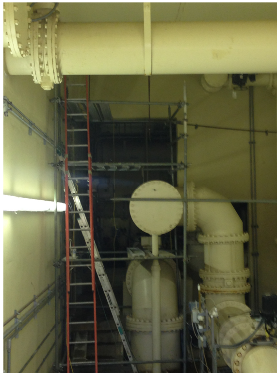
February 19, 2015 – Demolition of existing dehumidifier in the pipe gallery
