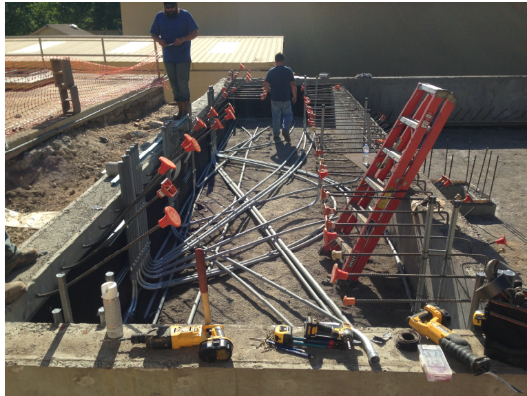
May 1, 2015 – Installing the new electrical conduit under the proposed floor slabs of the new alum building and stub up above FFE.
