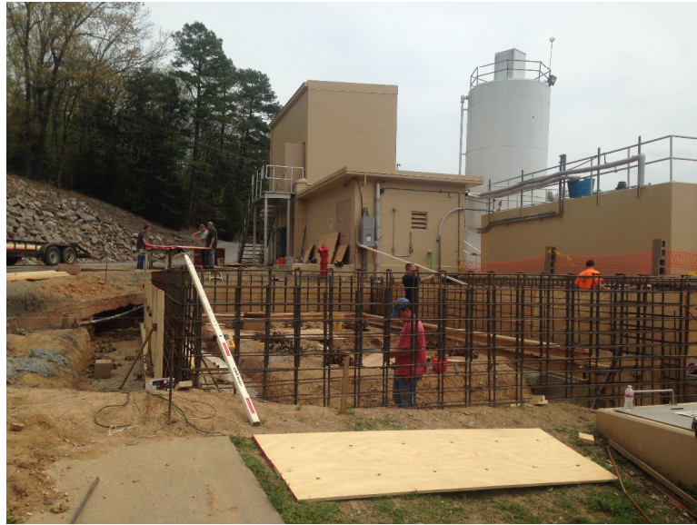
April 8, 2015 – Placing concrete forms for the construction of the foundation stem walls.
