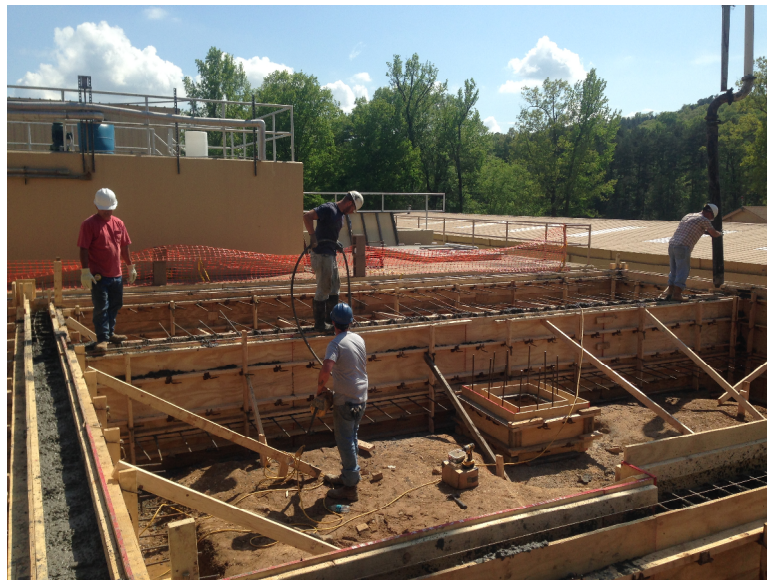
April 17, 2015 – Placing concrete with pump truck.
