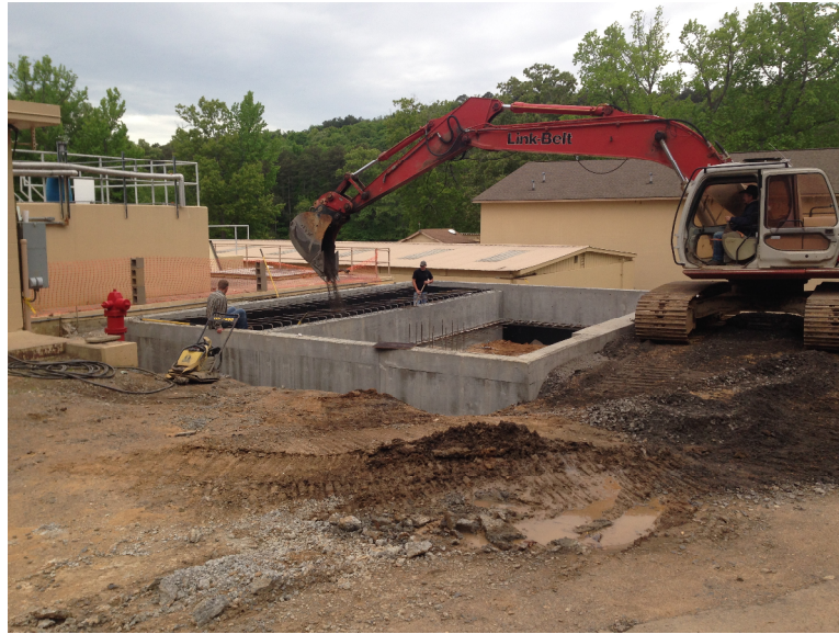
April 27, 2015 – Place compacted select class 7 stone backfill around the outside of the new alum building foundation stem walls.
